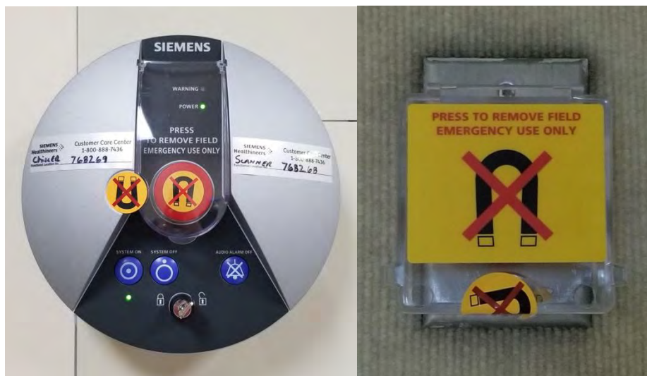
Figure 11: At left, the Control Room quench button in red, with yellow sticker and plastic shielding. At right, the Scanner Room quench button in yellow.
